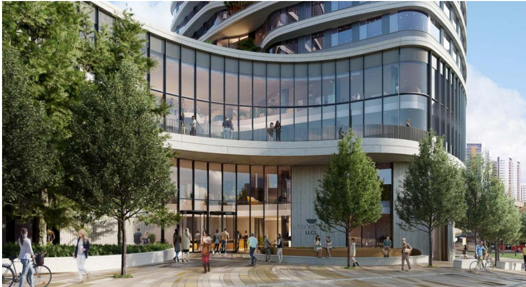
Figure 6 - Main Student accommodation entrance along Trafalgar Way
